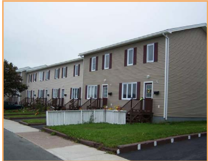
Salter Place modernization
